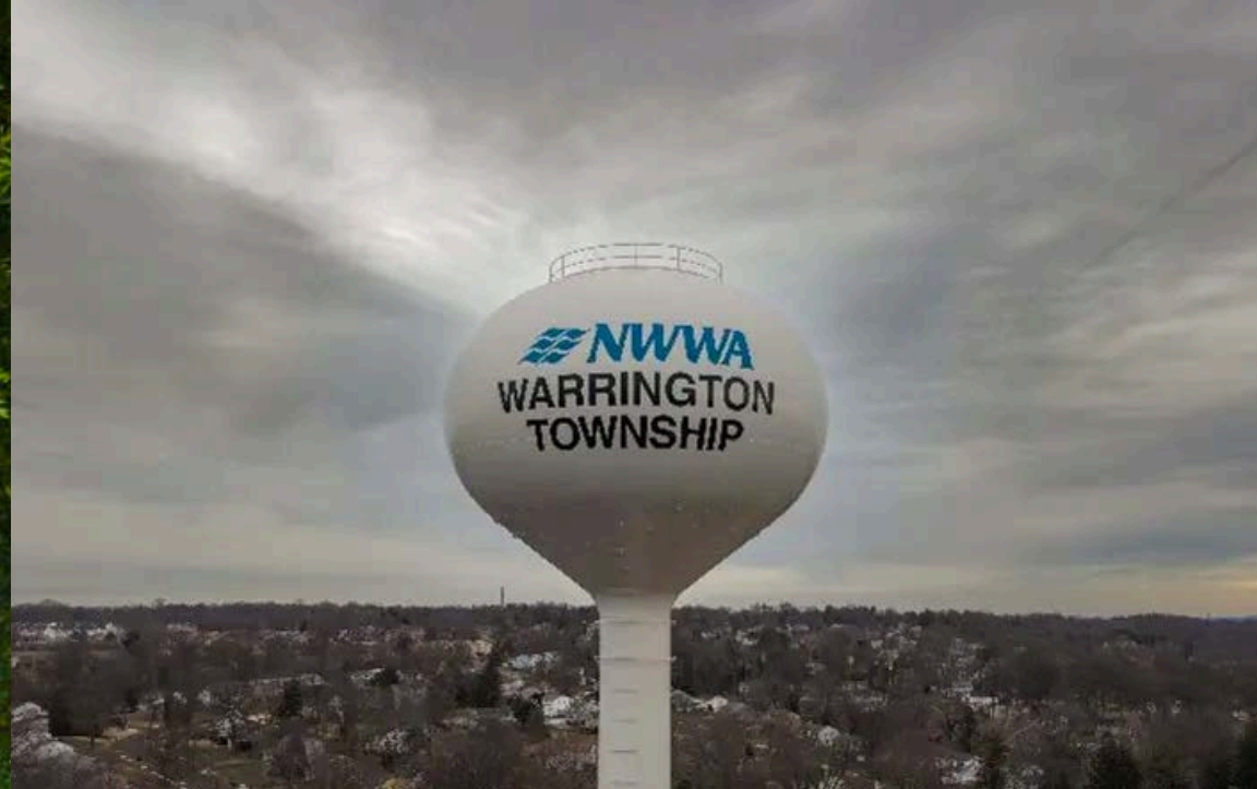
SHETLAND TANK MAINTENANCE AND IMPROVEMENTS - $1,000,000 Warrington Township, Bucks County, PA
