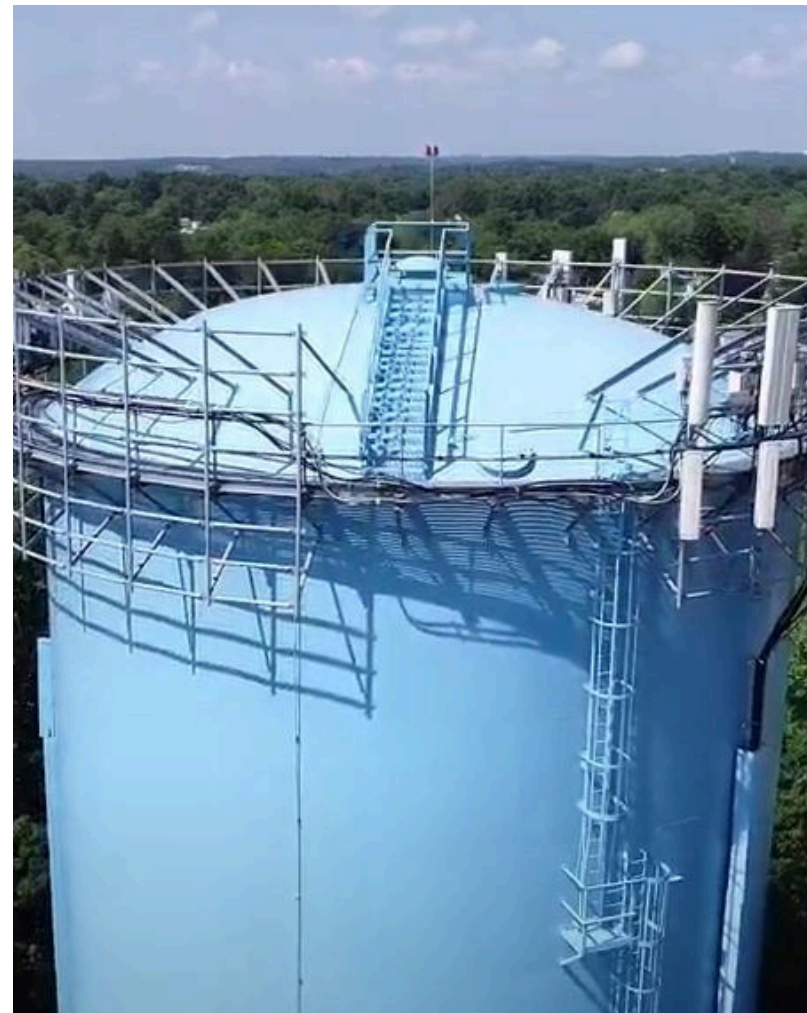
FEASTERVILLE WATER TANK Lower Southampton Township, Bucks County, PA
