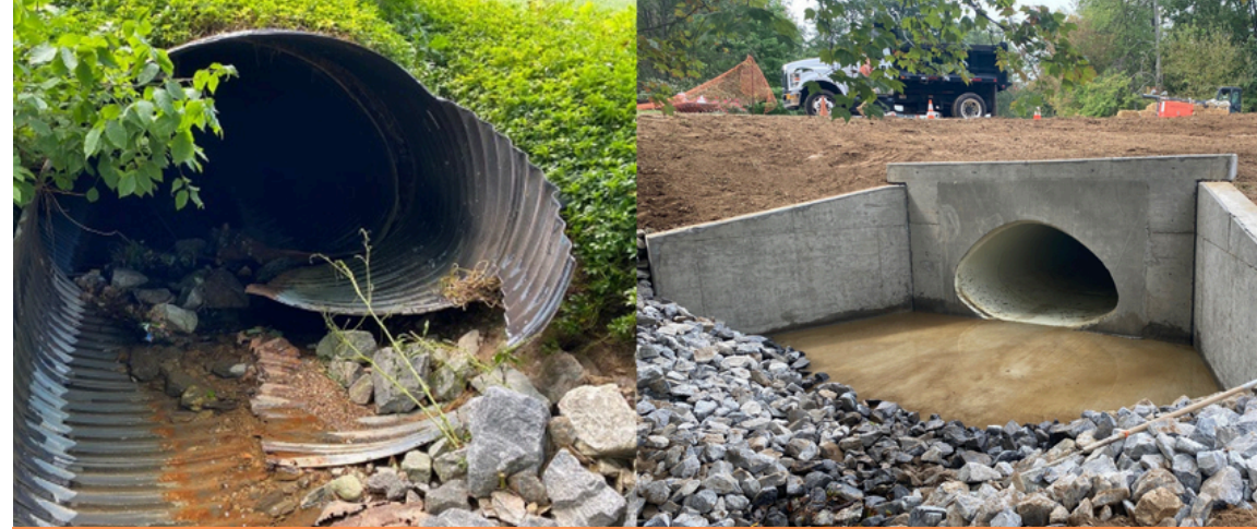
KNOLLWOOD DRIVE CULVERT REPLACEMENT West Goshen Township, Chester County, PA
