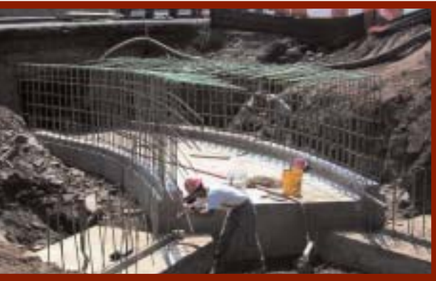
Meetinghouse Road box culvert
